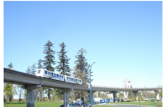
Figure 3: AGT/Elevated LRT: The Vancouver SkyTrain
